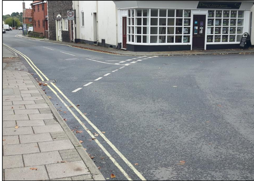
Figure 3-2 Low kerb heights and building thresholds on Valley Road
