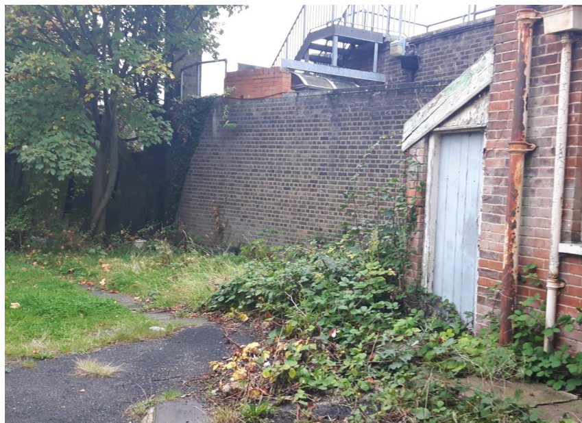
Figure 3-4 Large wall in car park east of High Street.
